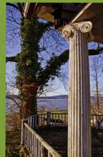
Punishing winter storms severely damaged the wooden columns and plaster capitals (right and above) around the house. "If it's possible to repair and reuse, I'll always choose that route," Tilly says. He consulted a master craftsman in nearby Yonkers, N.Y., who made a mold and cast new capitals. Contractors scraped, primed, and reinstalled the columns (left).
