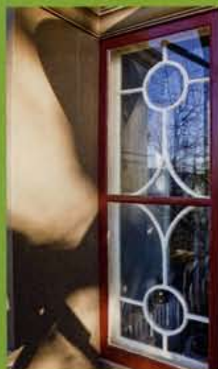
Greening the 1904 cottage meant reusing existing treasures, and replicating others with sustainable materials. Tilly repaired and rehabilitated the sidelight and a wooden storm window flanking the front door (left). Instead of tearing out damaged flooring, he and Martin had original floors sanded and refinished (middle). Historically appropriate cedar shingles (right) replaced asphalt shingles on the roof.
