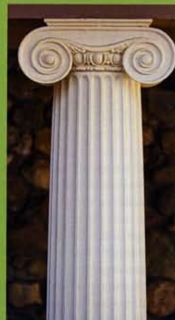
Punishing winter storms severely damaged the wooden columns and plaster capitals (right and above) around the house. "If it's possible to repair and reuse, I'll always choose that route," Tilly says. He consulted a master craftsman in nearby Yonkers, N.Y., who made a mold and cast new capitals. Contractors scraped, primed, and reinstalled the columns (left).
