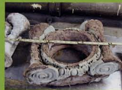
Punishing winter storms severely damaged the wooden columns and plaster capitals (right and above) around the house. "If it's possible to repair and reuse, I'll always choose that route," Tilly says. He consulted a master craftsman in nearby Yonkers, N.Y., who made a mold and cast new capitals. Contractors scraped, primed, and reinstalled the columns (left).
