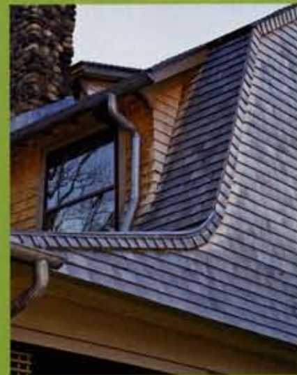
Greening the 1904 cottage meant reusing existing treasures, and replicating others with sustainable materials. Tilly repaired and rehabilitated the sidelight and a wooden storm window flanking the front door (left). Instead of tearing out damaged flooring, he and Martin had original floors sanded and refinished (middle). Historically appropriate cedar shingles (right) replaced asphalt shingles on the roof.
